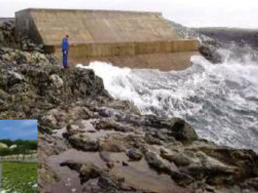
LIMPET (Land Installed Marine Power Energy Transmitter Islay – Scotland (500kW) 2000
